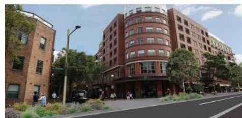
PROPOSED VIEW: View north-west towards intersection of Crown Street and Fitzroy Street
